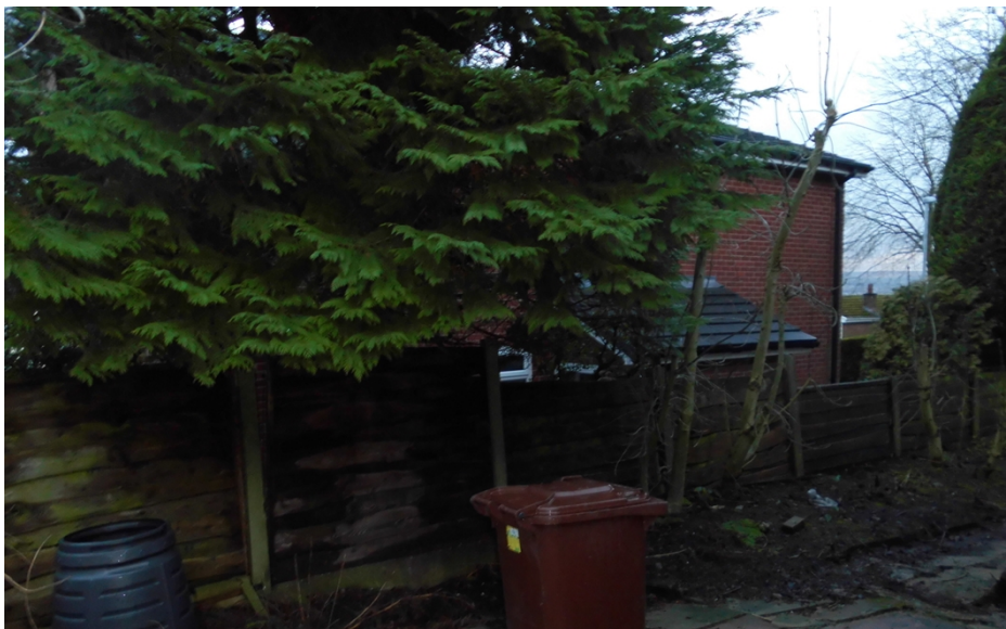
Rear of 2 storey extension
