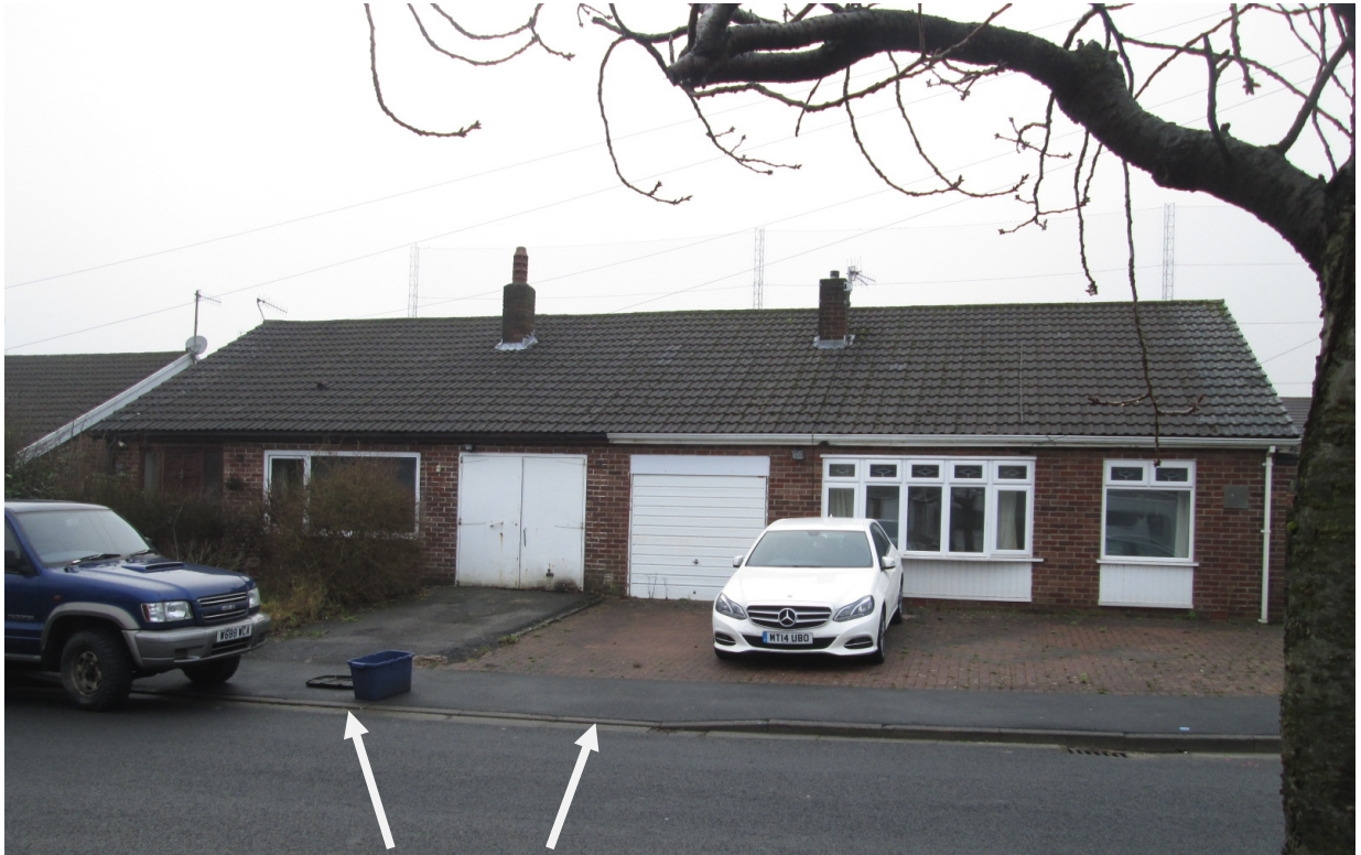
nos. 46 and 48 Lindale Crescent ( as existing)
